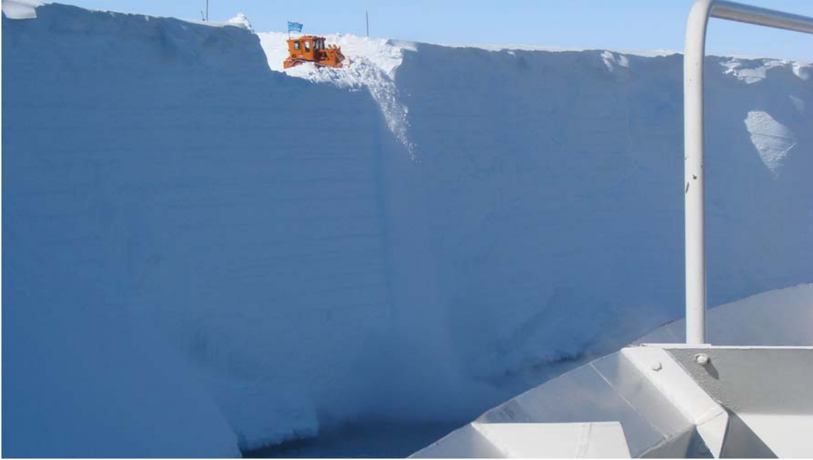
“A Bulldozer busy preparing the ramp for off-loading of cargo”
